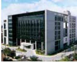
Taoyuan Technology Center (Green Building)
